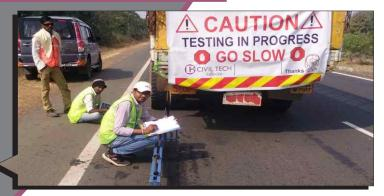
This method of test covers determination of pavement and existing flexible surface and to get information about the overlay design (Crust Thickness).
